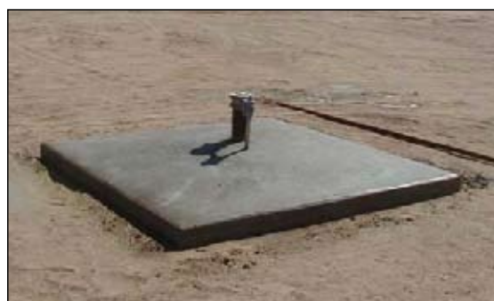
Example of a properly protected wellhead.
