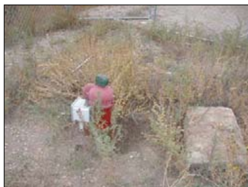
Another example of an unprotected wellhead.
