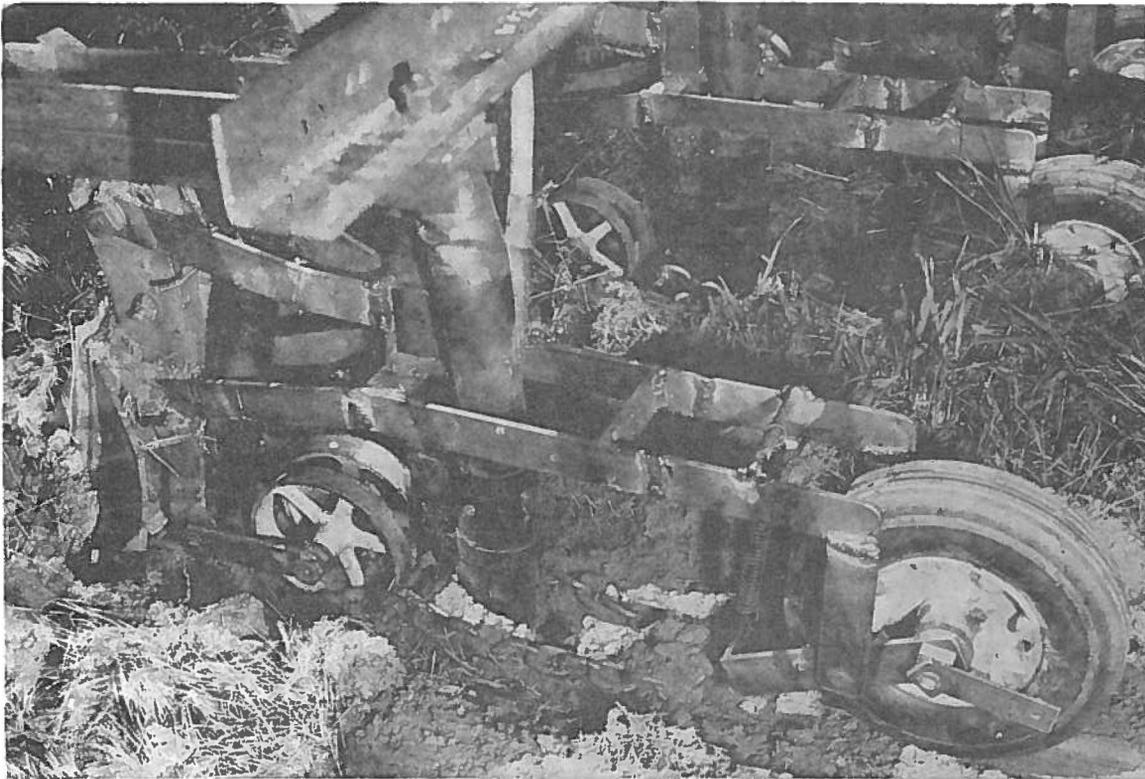
Left to right: Lister blade, fertilizer tube, split press wheel, seed tube, drag chain and final press wheel.
