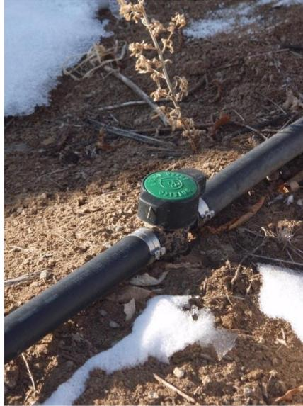
Fig. 2 Valves used to isolate RDI trees from irrigation during Phase II at the Mesa site.
