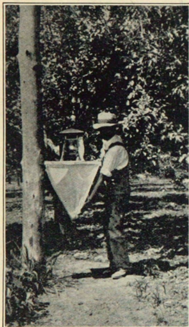
Fig. 4.—Electrocutor style of trap and cheese-cloth funnel as used in an experimental test in A. L. Roberts' orchard.
