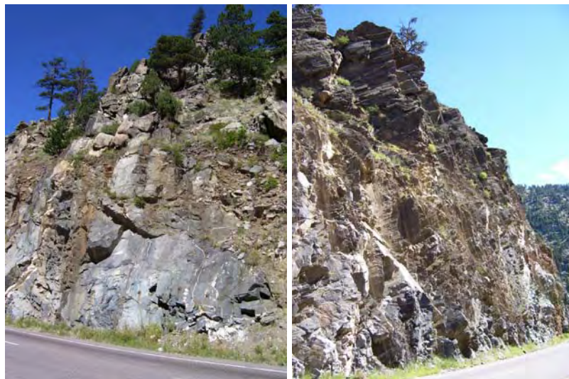
Figure 2.35: Example of mitigation effectiveness graded as D: Picture was taken on CO 14 in Larimer County. Mitigation consisted of mesh. The mesh is confined to only one section of the slope. Large blocks can easily dislodge and would likely tear the mesh from the slope.
