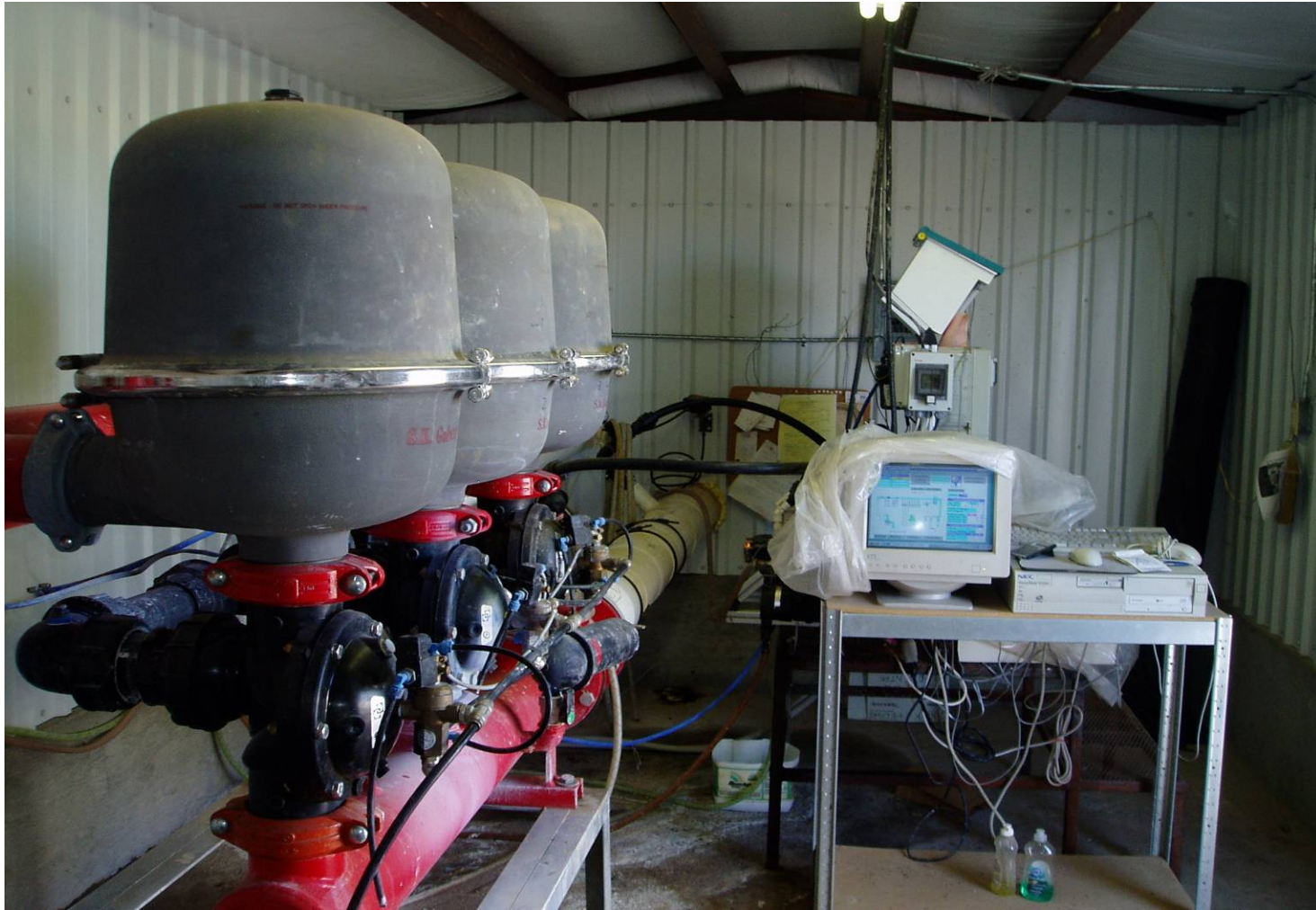
Picture 2. Computer control and filters for drip system.
