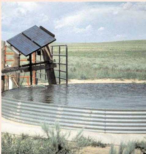
This portable PV system pumps 1.75 gallons per minute from a 60-foot well to fill a remote stock tank.
